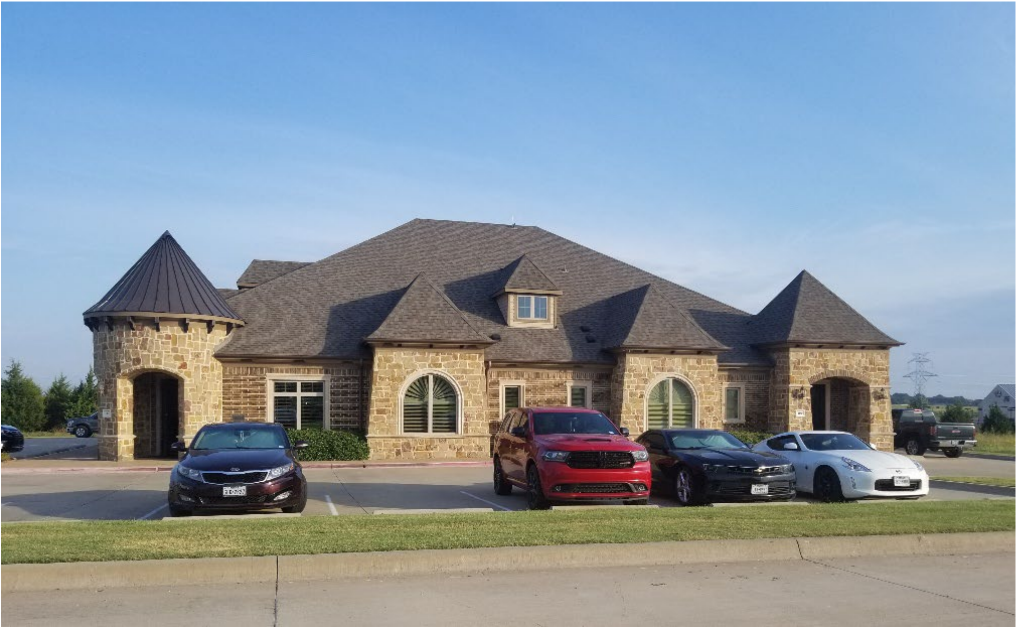
Existing office building.
