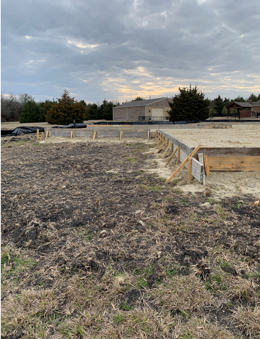
Looking northwest along the forms at the rear of the form boards
