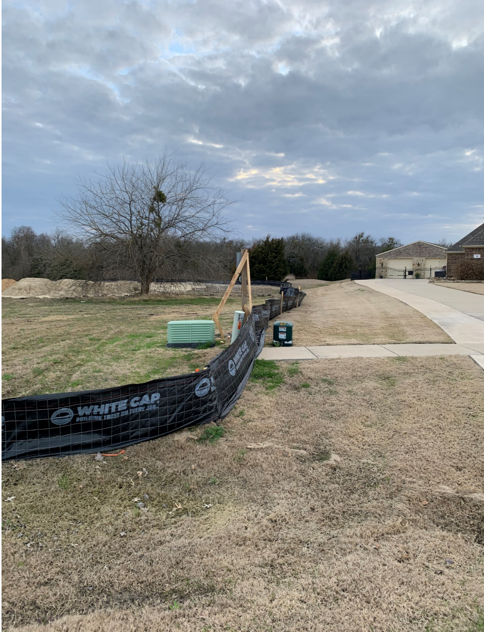
Looking down the southwest property line from Fireside Drive
