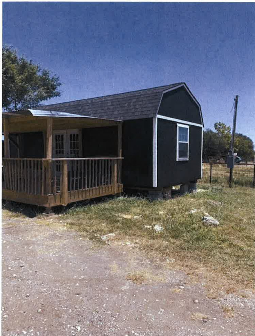
View of accessory structure looking easterly from subject property
