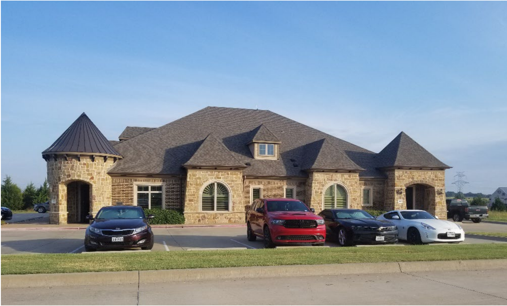
Existing office building.
