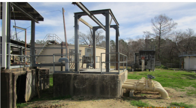
City of Kirbyville, DR WWTP Improvements
