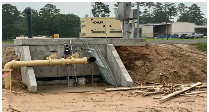
City of Kirbyville, DR Sewer Improvements
