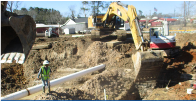
City of Kirbyville, DR Drainage Improvements
