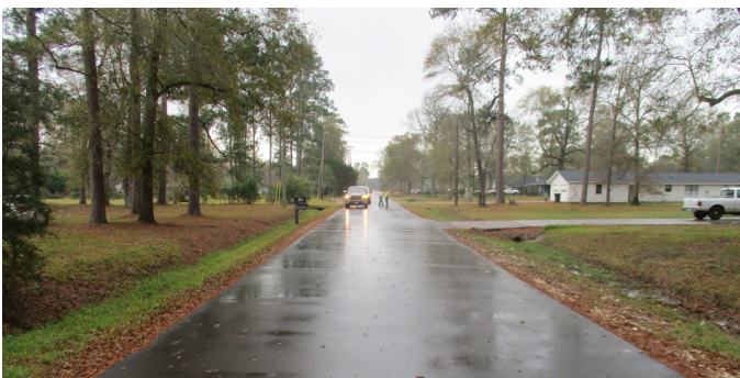
City of Vidor, FEMA Street Improvements
