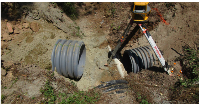
City of Lumberton, DR Drainage Improvements
