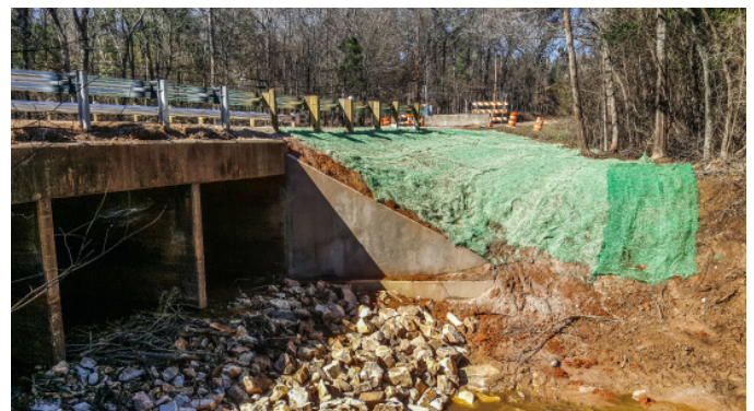
City of Kilgore, FEMA Wingwall Rehabilitation
