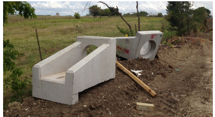
City of Terrell, FEMA CR 305 Rehabilitation
