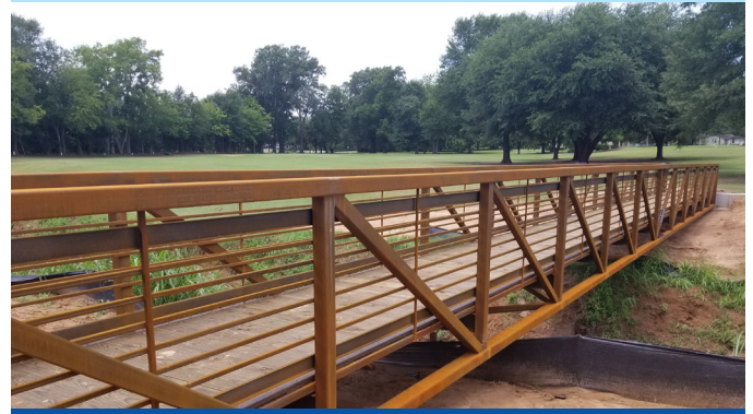
City of Kilgore, FEMA Replacement of Pedestrian Bridges
