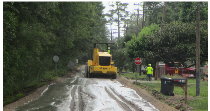
City of Pinehurst, DR Street Improvements
