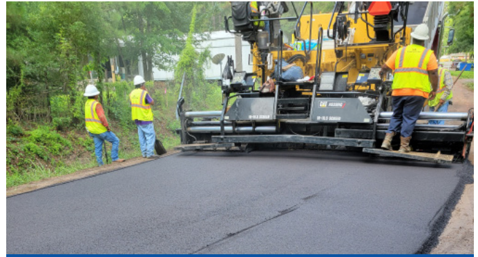
City of Lumberton, DR Street Improvements
