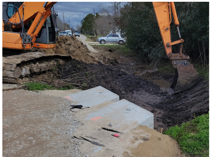
Galveston County Algoa Alto Loma Culvert Replacement
