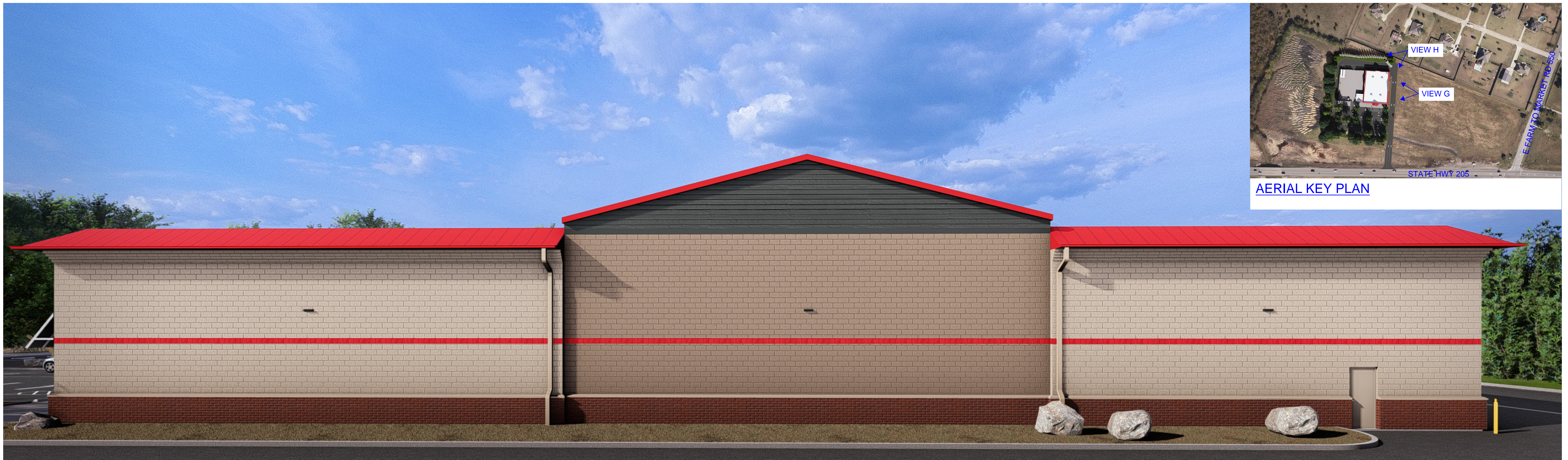
VIEW G: RIGHT SIDE OF BUILDING
