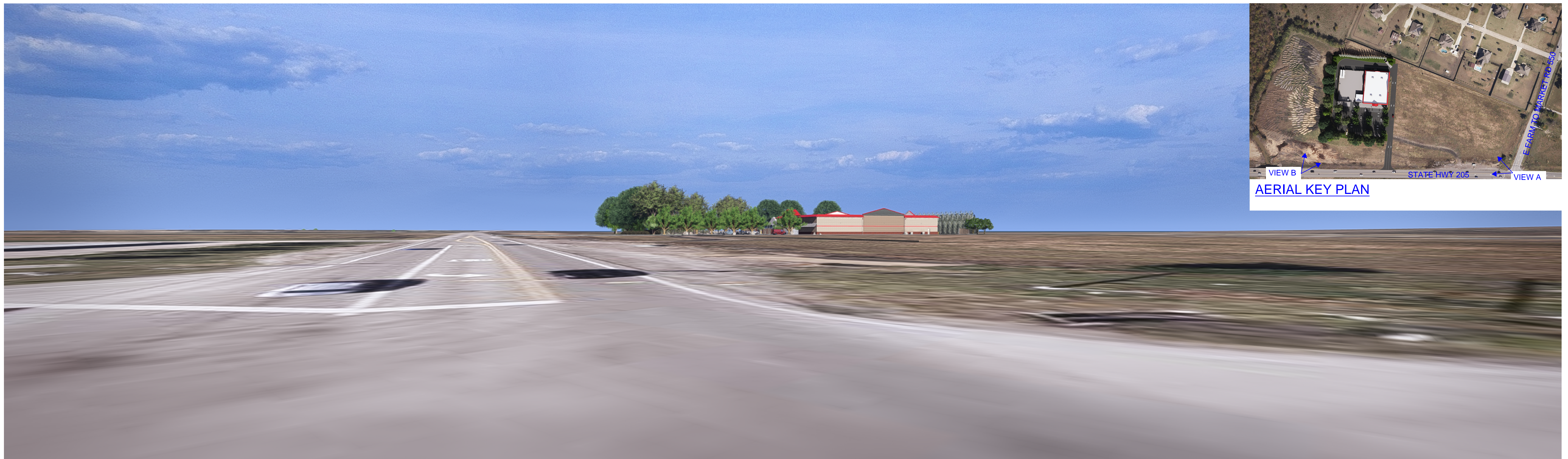
VIEW A: NORTH-WEST FROM E FARM TO MARKET RD 550 / STATE HWY 205
