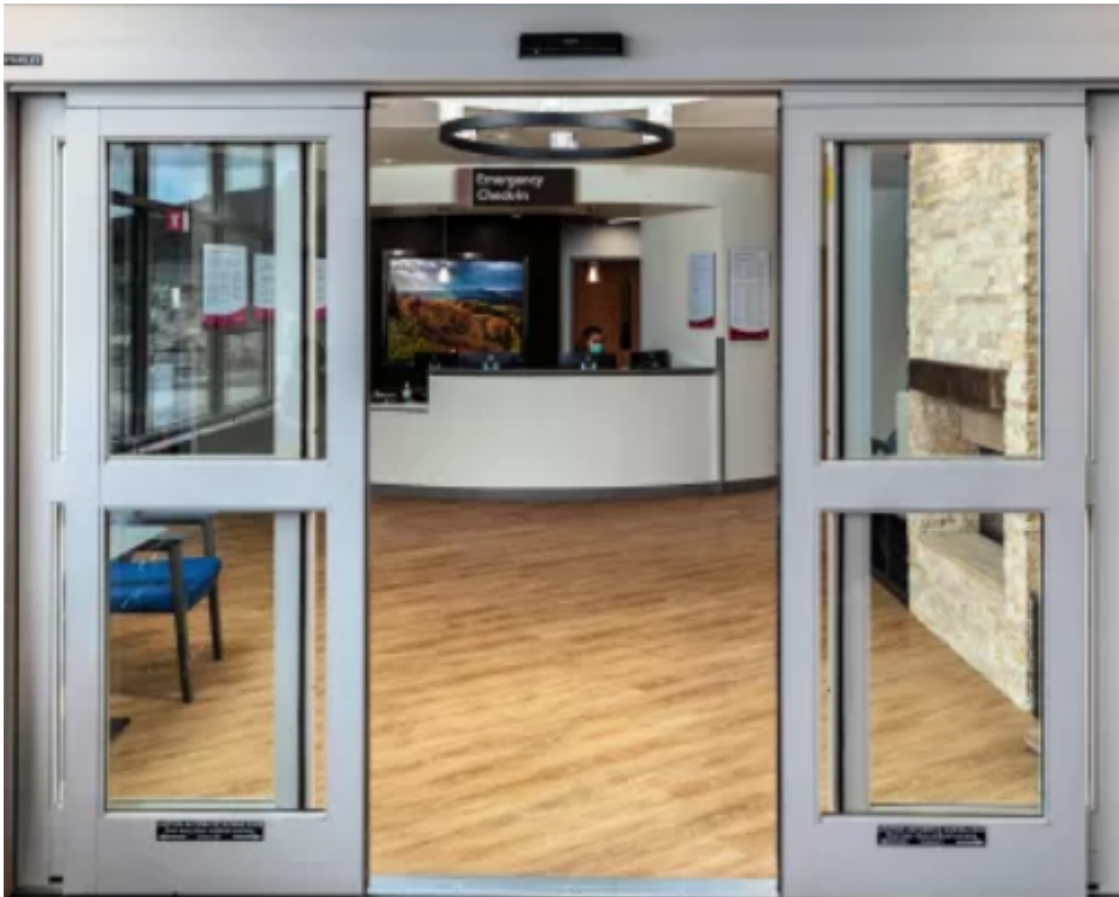
SOREFRONT SYTEM AND ENTRY DOOR MANUF: STANLEY COLOR: ANDOZIED ALUMINUM
