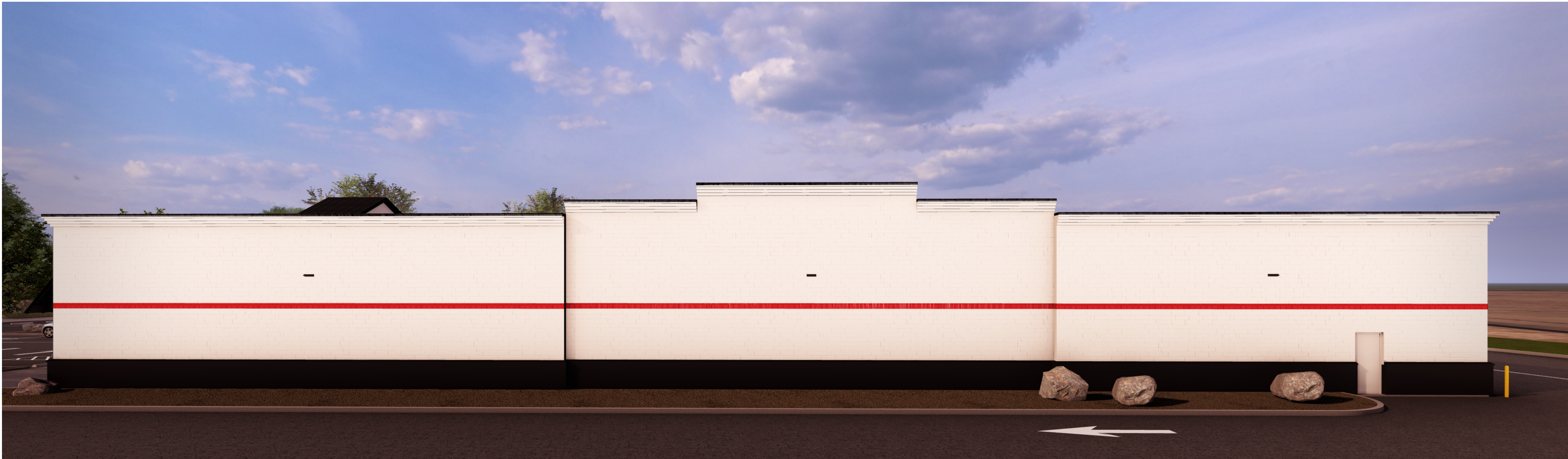
VIEW F: RIGHT SIDE OF BUILDING
